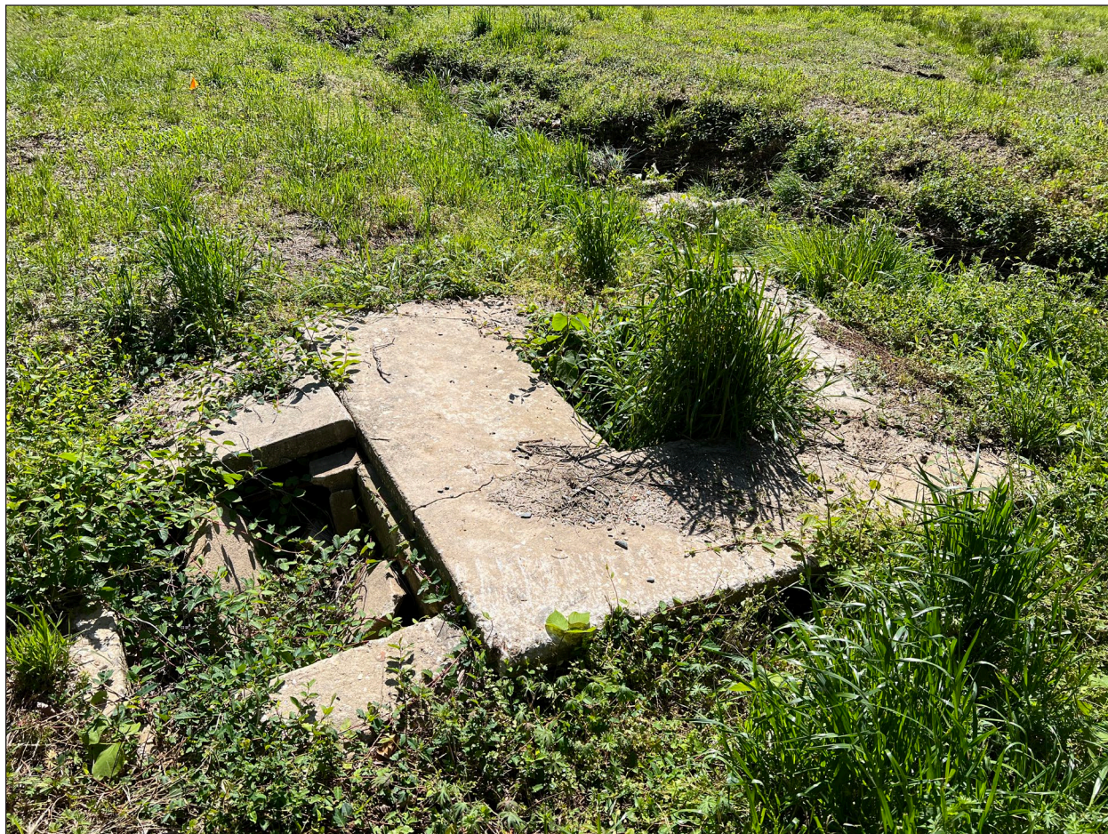
Figure 15. Feature 2 - The Concrete Foundation, Facing Southeast
