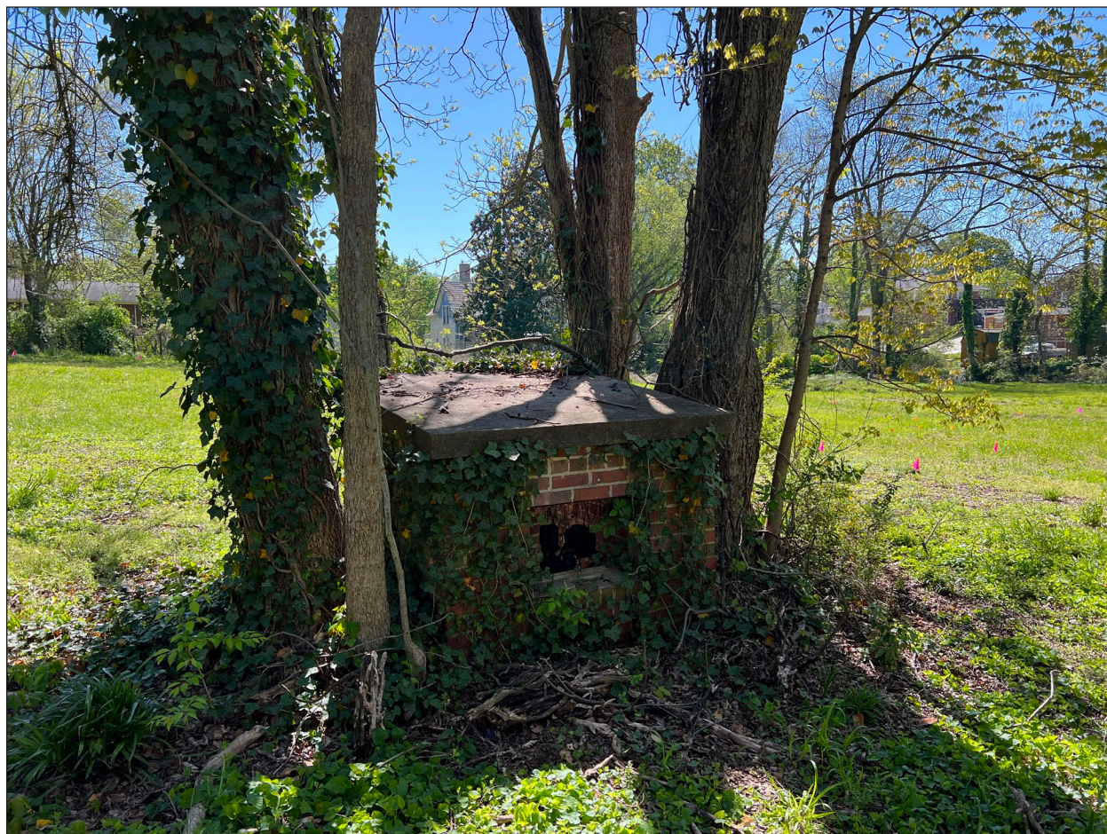
Figure 14. Feature 1 - The Brick Utility House, Facing Southeast
