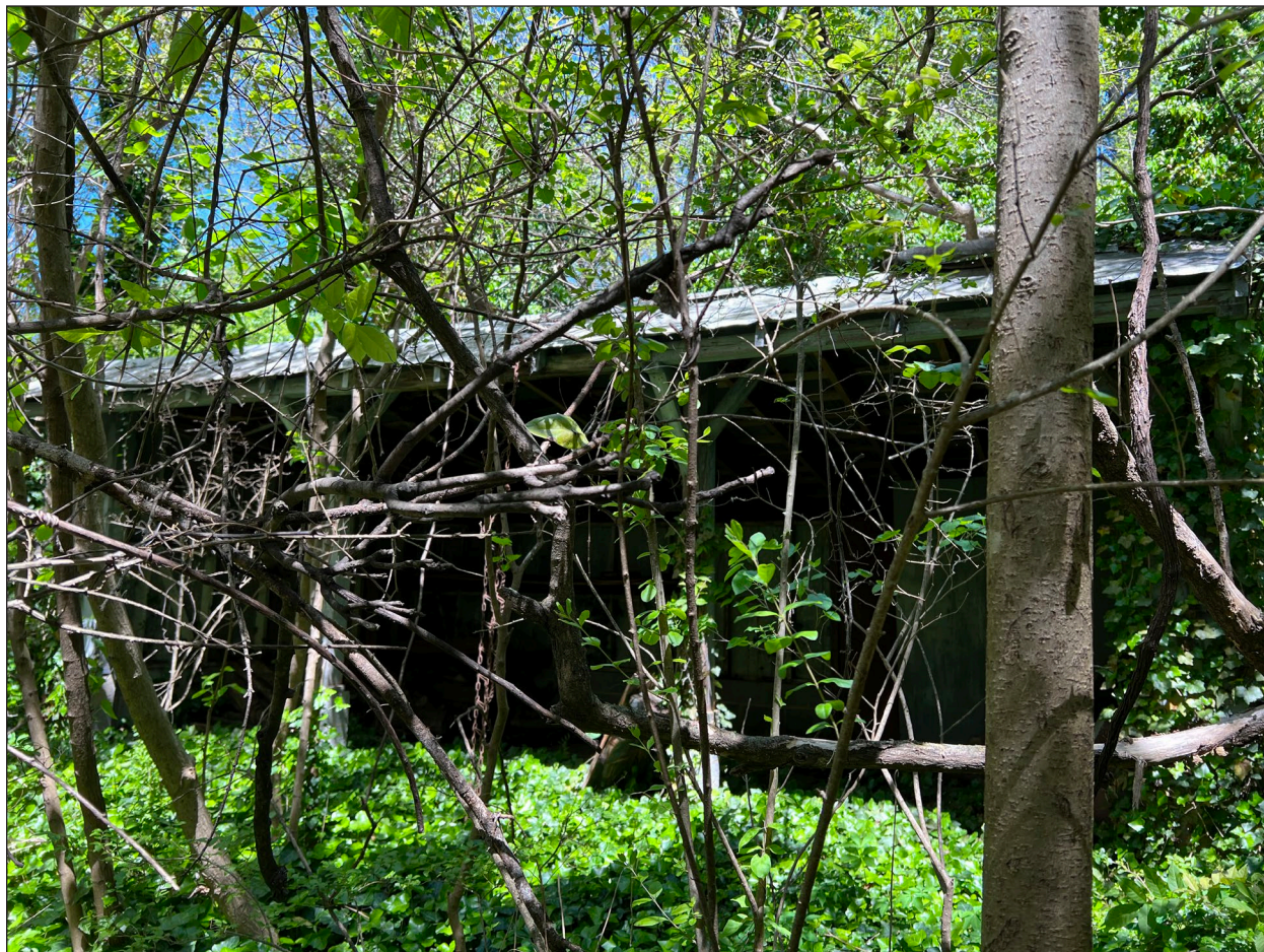
Figure 16. Feature 4 - The Modern Agricultural Shed, Facing North
